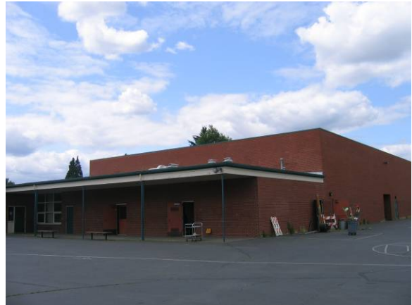
South elevation facing northwest
