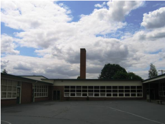
East elevation facing northwest
