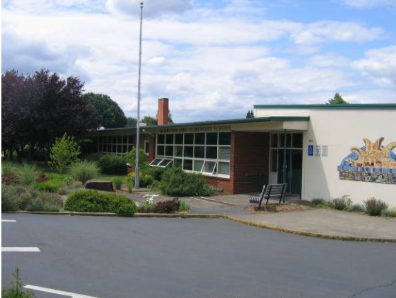
South elevation facing west
